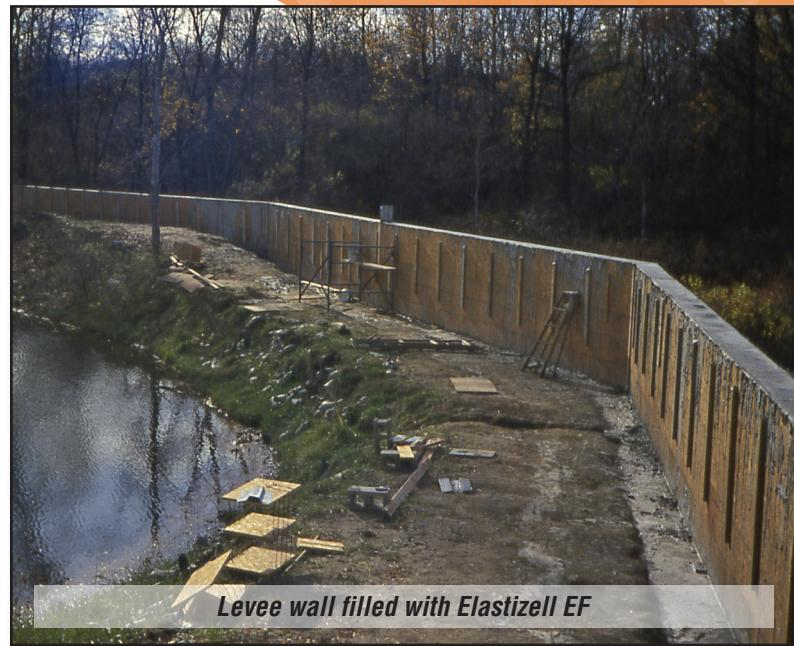
Levee wall filled with Elastizell EF
